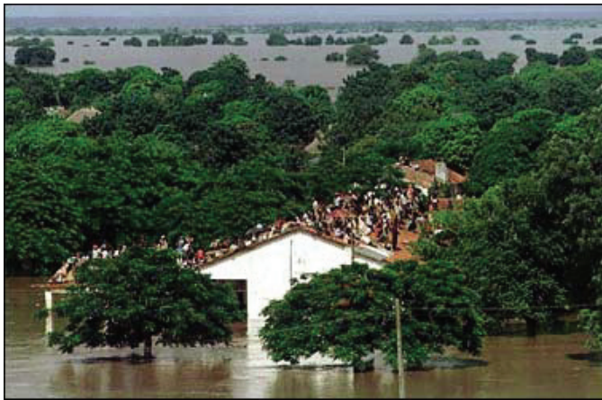
FIGURE 11.2.2 The Mozambique flood of 2000 flooded over 19,000 square miles at its maximum and damaged as much as 90 percent of the country's irrigation infrastructure. Some 45,000 people were rescued from rooftops. SOURCE: AP/Wide World Photos.
